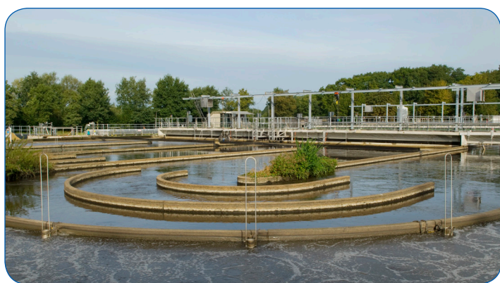
An example of a water resource recovery facility.
